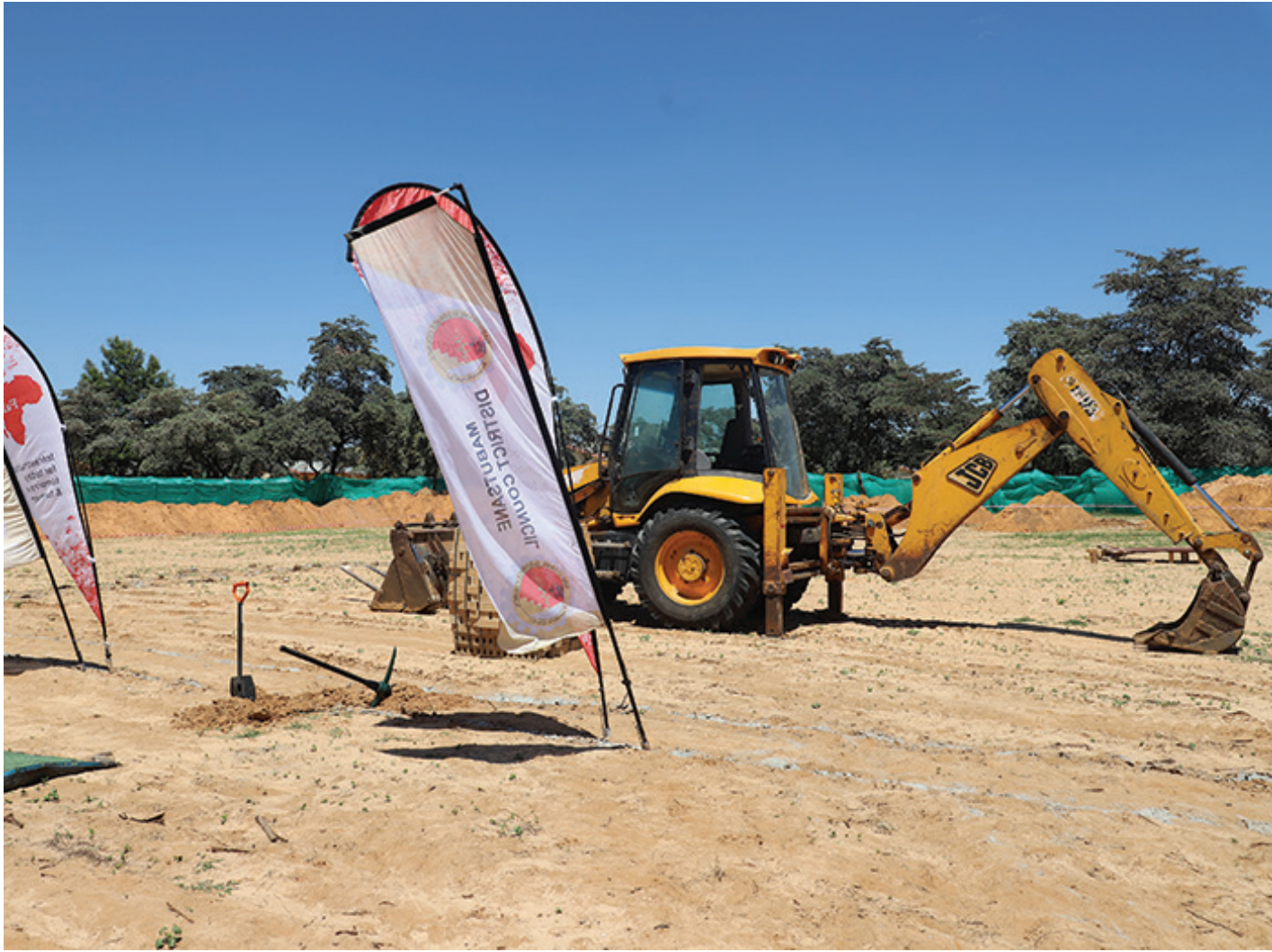
Project Construction Site
